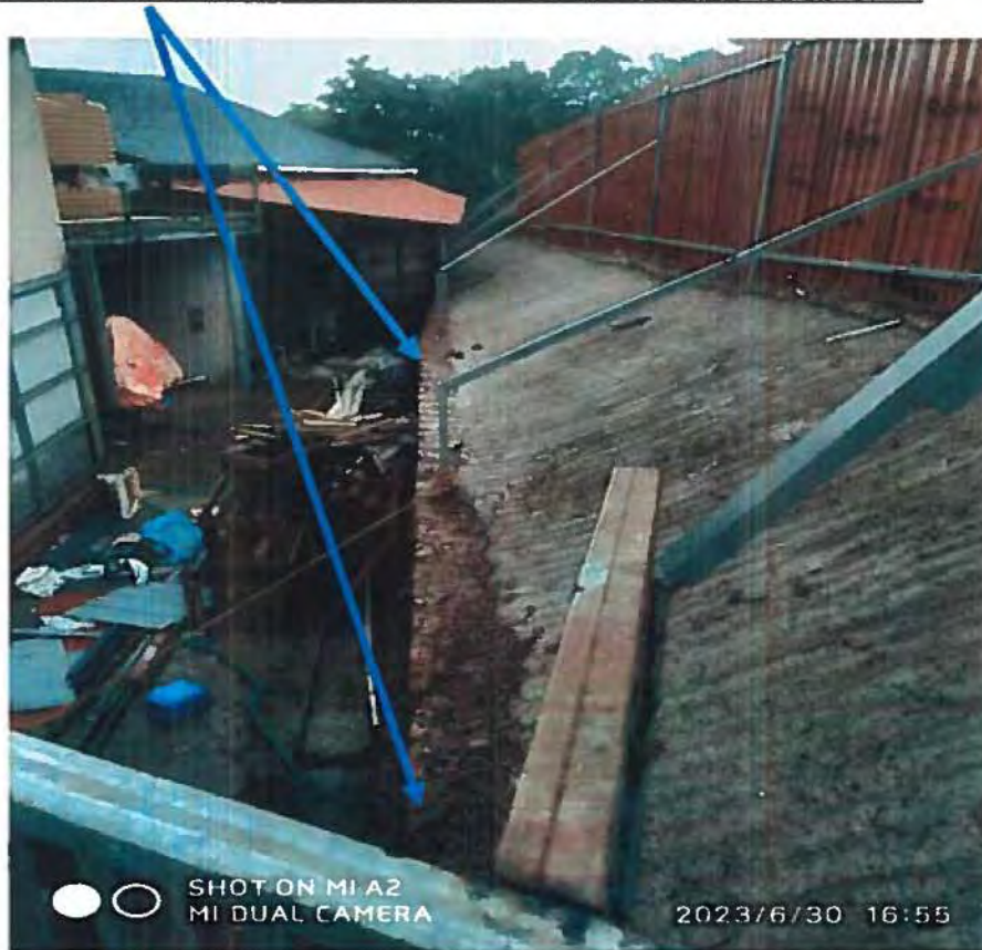
LATERITE STONE RETAINING WALL BETWEEN NORTHERN SIDE BOUNDARY AND STRUCTURE 'I'.
