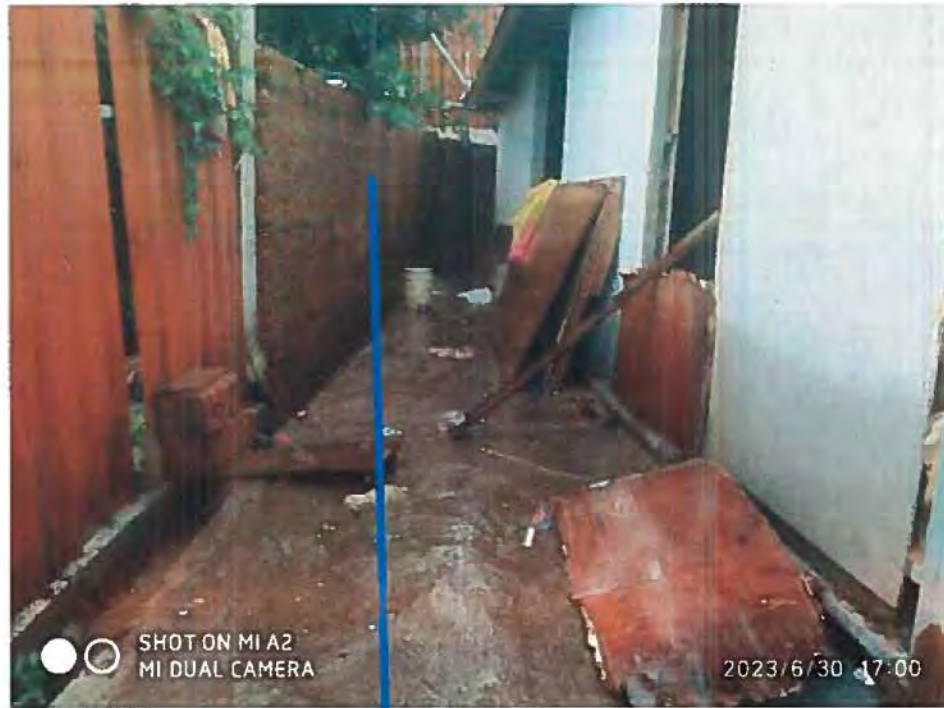
CONTINUATION OF RETAINING WALL NORTH-EAST SIDE OF LAND IN QUESTION.
