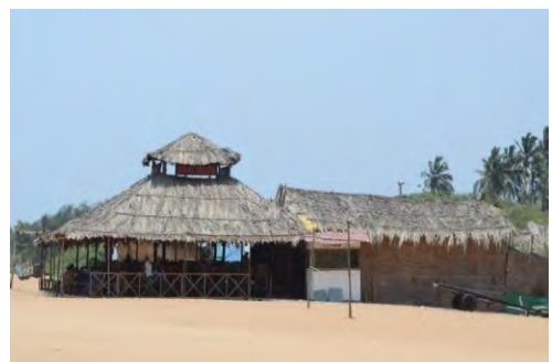
Figure 1: Beach Shacks, Goa
